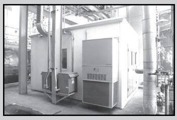
Temperature controlled, sound attenuating panel construction protects computer systems used in the manufacture of electric power.
