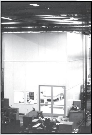
Temperature gradient within 20'-0" cleanroom is maintained at  $\pm$  1° F over one meter.
