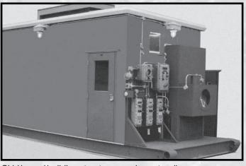
Skid based building structures enclose standby or emergency power generators, compressors, and communication equipment.
