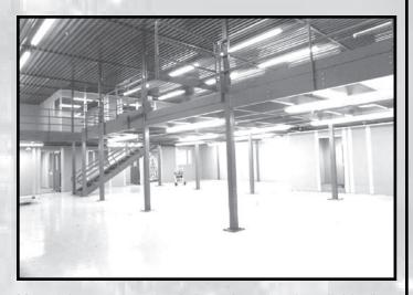
Mezzanine structure optimizes the use of available floor space permitting the installation of offices and laborato-
