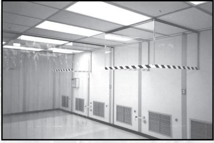
Multiple cleanroom classifications are established within the same building envelope utilizing clear vinyl softwall panels.
